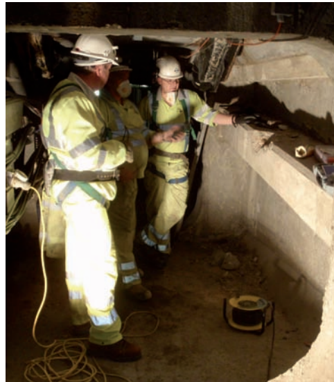
Left: Carrying out the blind wire test. Right: Total station prisms inside the box monitor movement.
